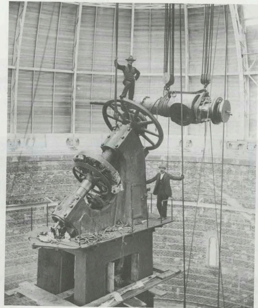
Hoisting the polar axis for the 40-inch Refractor, 1896.
