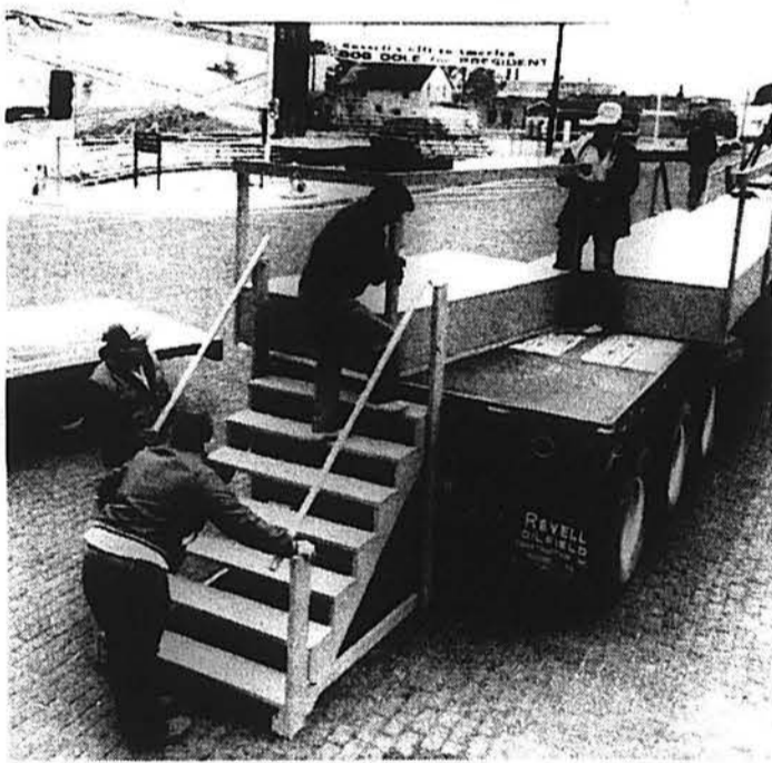
Workers installed platforms Sunday upon which the press will stand when Dole announces his campaign this morning in Russell.
