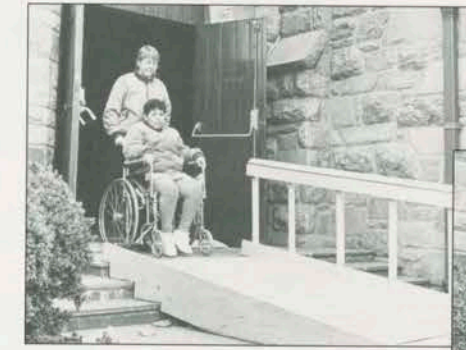
Build a ramp for wheelchair use and everyone benefits.
