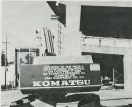
Two hydraulic excavators were donated by Komatsu Dresser to work on the collapsed Cypress structure of Interstate 880 in Oakland following the recent earthquake.
